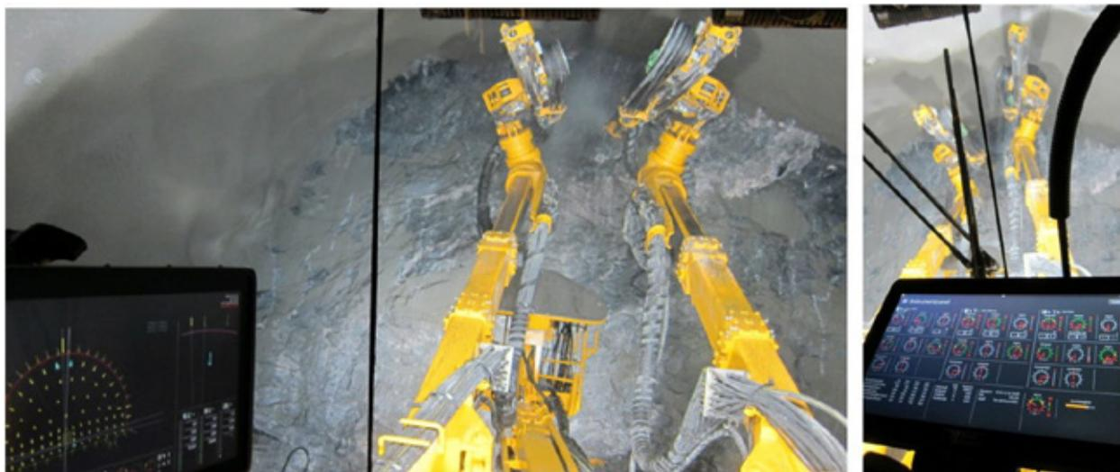
Figure 1.3.1: Bever controls computerized drill system mounted on a drill rig. The screen to the left displays the drill plan, the screen shows which holes are currently being drilled (highlighted in blue). The screen to the right is the instrumental panel and shows a detailed view of all the parameters for each boom.
