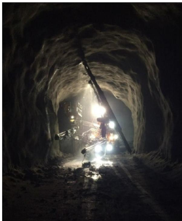
Figure 1.3.23: Jumbo drilling bolt holes.
