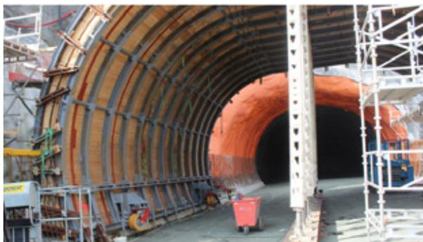
Figure 1.4.1: Formwork wagon from Alsaker.
