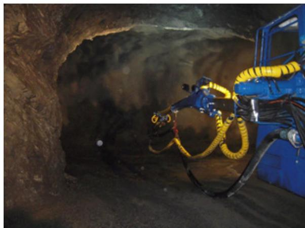
Figure 1.3.18: Shotcrete rig the tunnel, ready for applying shotcrete on the rock surface.
